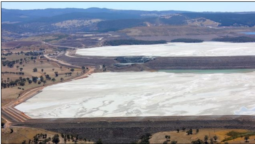
Figure 3 The tailings dam failure at Cadia mine in Australia. Image from Newcrest.
